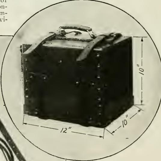
One of the Latest Compact Radio Sets Designed Especially for Field Military Service. It Has a Powerful Transmitter Operating on a Storage or Dry Battery.
