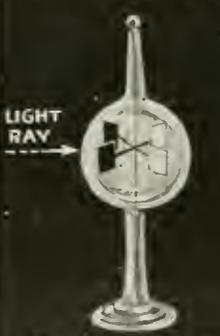
*The pressure of light has been measured. It will spin the vanes of the radiometer.*
