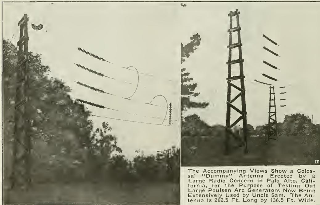
The Accompanying Views Show a Colossal "Dummy" Antenna Erected by a Large Radio Concern in Palo Alto, California, for the Purpose of Testing Out Large Poulsen Arc Generators Now Being Extensively Used by Uncle Sam. The Antenna Is 262.5 Ft. Long by 136.5 Ft. Wide.
